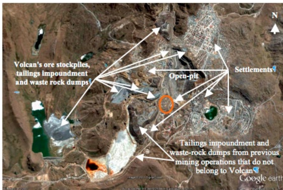
Figure 2: Google Earth satellite image of Cerro de Pasco. The open-pit mine and the company's tailings impoundment, waste rock dumps and ore stockpiles are marked, as are residential areas and dumps that do not belong to Volcan. The Ayapoto neighbourhood, which is mentioned later in this recommendation, is marked with a circle.
